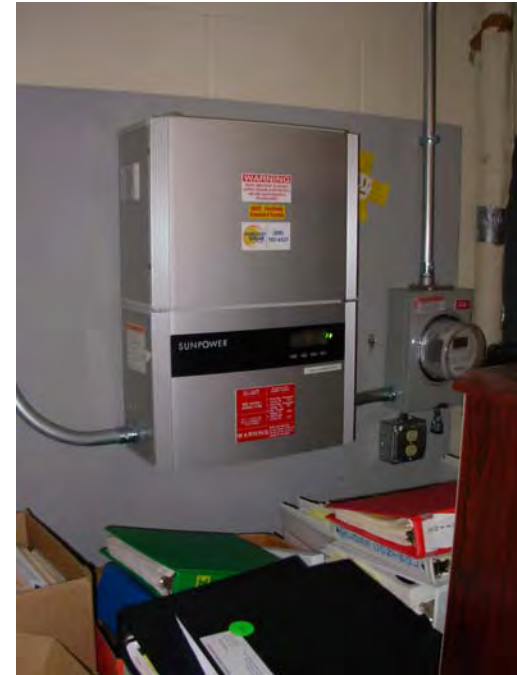
10. Inverters associated with solar panels
