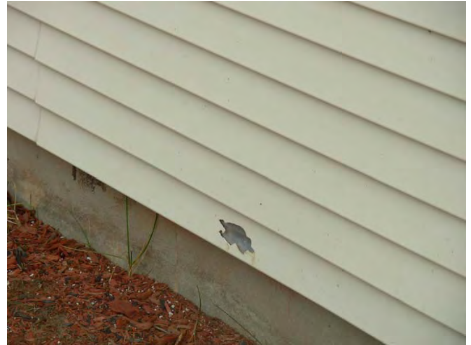
6. Spot vinyl siding damage
