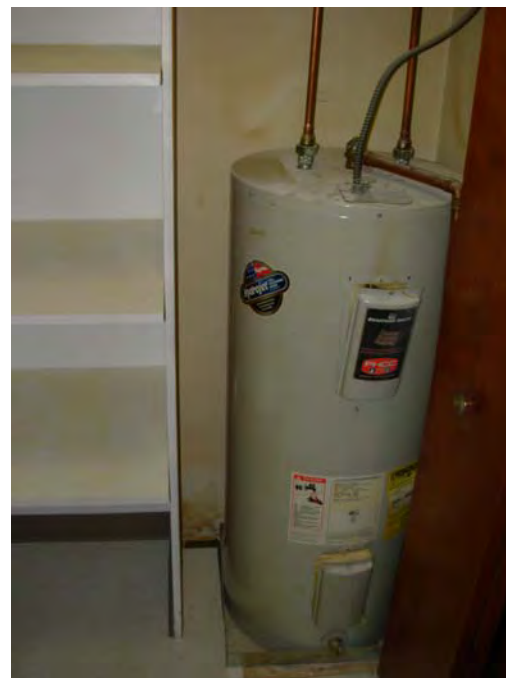
16. Typical domestic hot water tanks serving apartments
