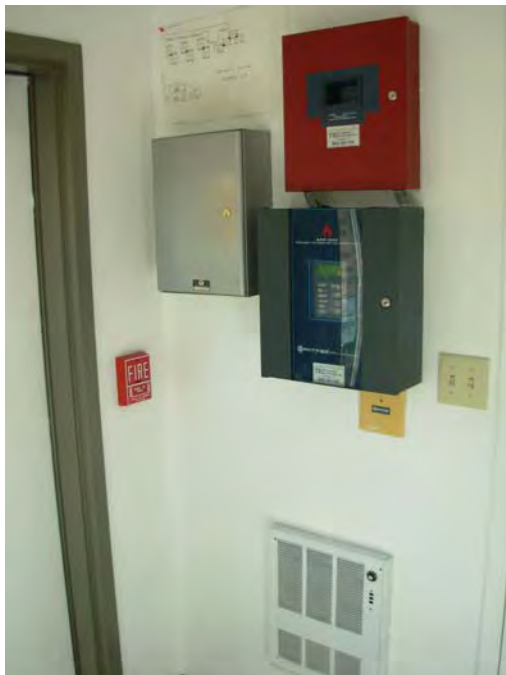
11. Fire detection - monitoring system serving property
