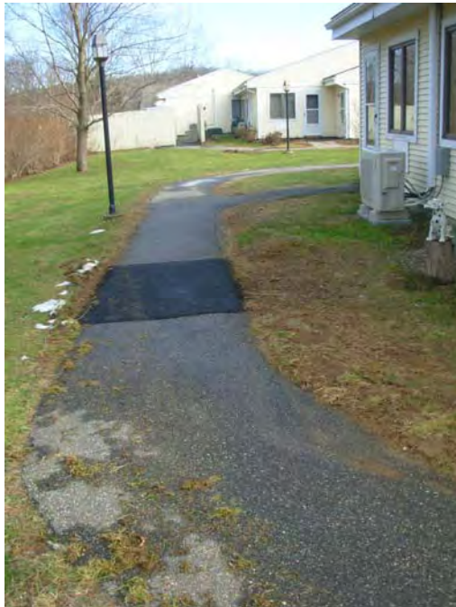
3. Recently patched walkway sections
