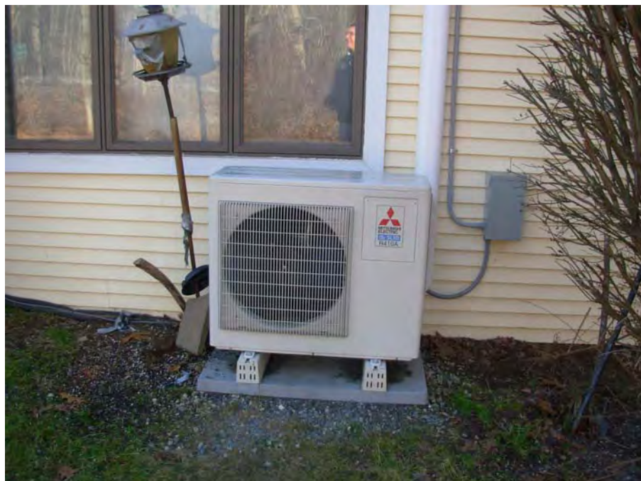
15. Unit heat pump exterior condenser unit
