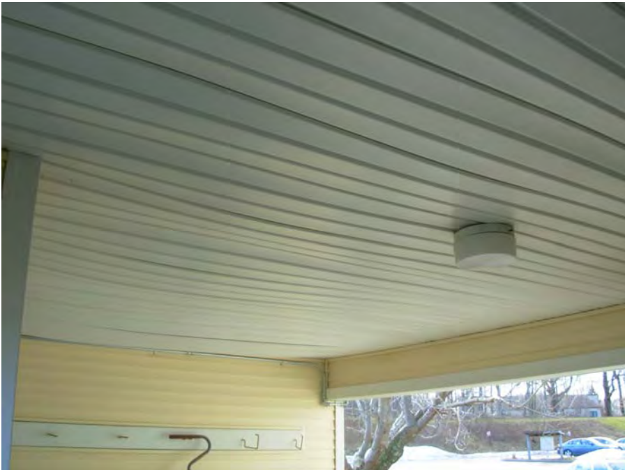
7. Sagging vinyl cladding at ceilings
